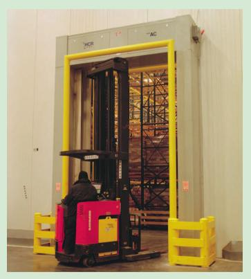
Freezer vestibules provide unrestricted doorway usage, are completely frost free, and ensure superior energy efficiency where conventional refrigeration is employed.
